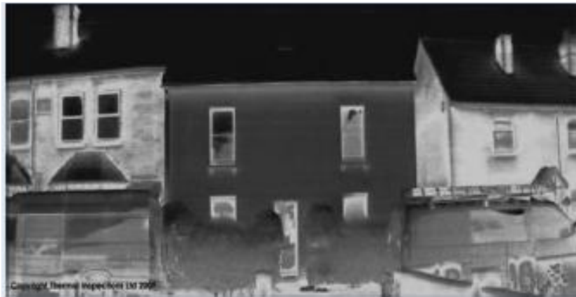
Fig. 11.3 Typical heat losses from an old domestic house.
